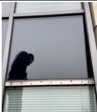
Opacified Glazed Spandrel (Type 2.1)
