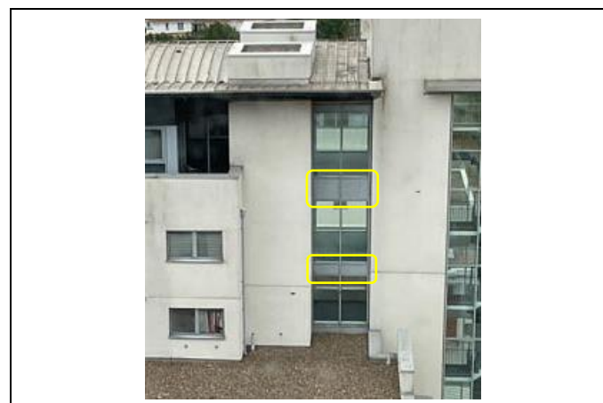
Figure 5 Typical Common Corridor Aluminium Spandrels (Panel Type 3.4)
