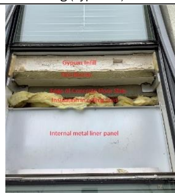
Exposed construction behind the glazed panel
