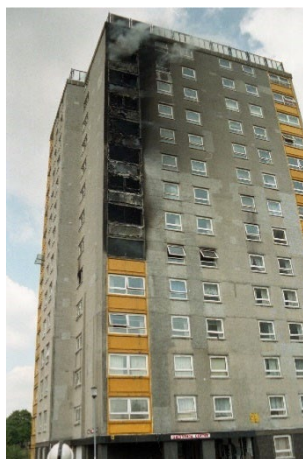
Figure D.3 – Fire at Garnock Court, Irvine
