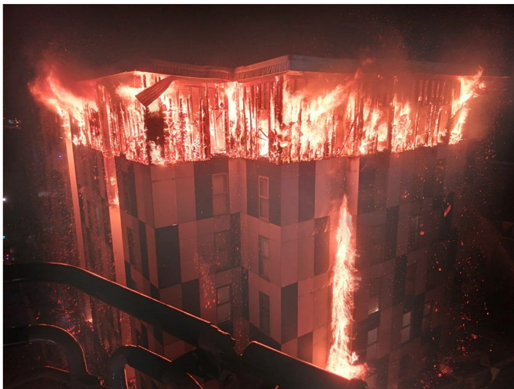
Figure D.6 – Fire at the Cube, Bolton
