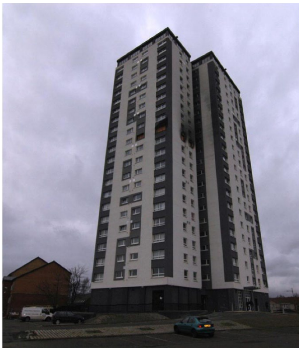
Figure D.7 – Fire in block resulting in limited external spread
